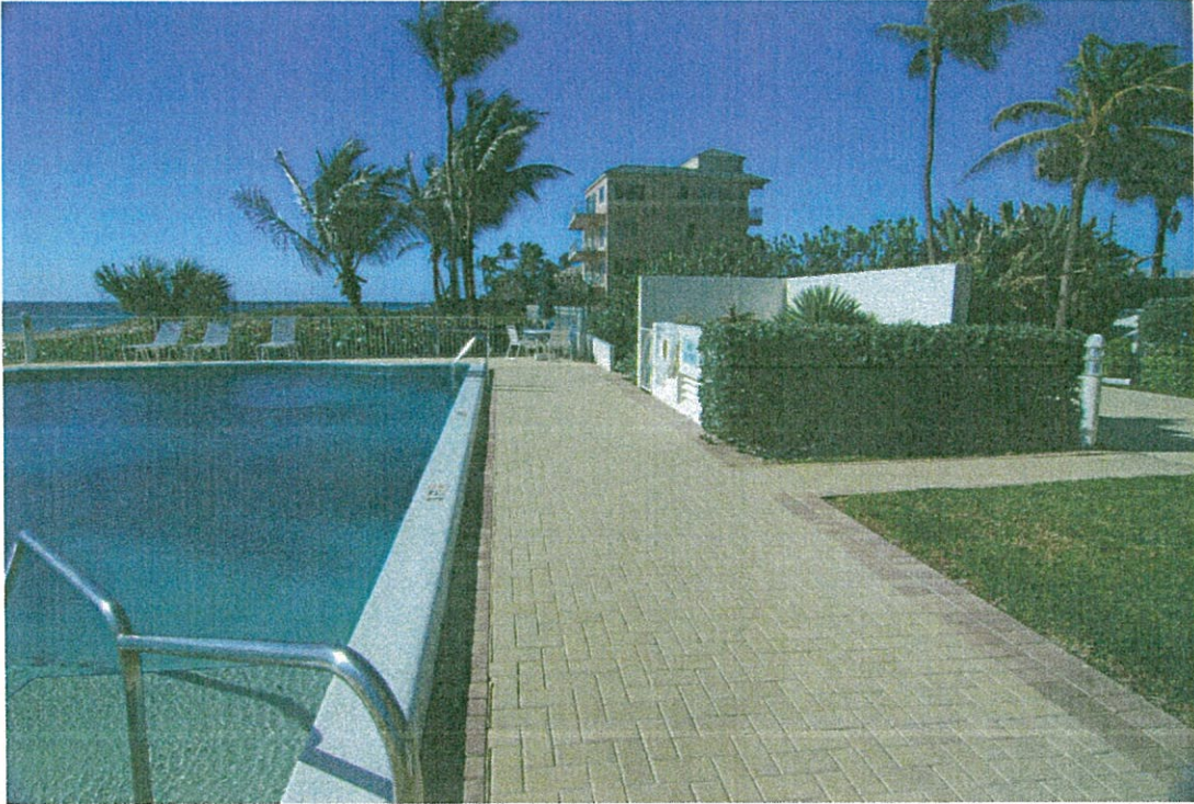
EXHIBIT 11. VIEW OF POOL, DECK AND POOL EQUIPMENT BUILDING LOOKING SOUTH
