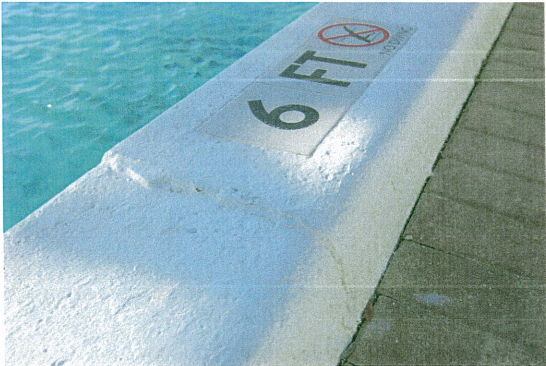
EXHIBIT 8. VIEW OF REPAIRED DISBONDED COPING STONE
