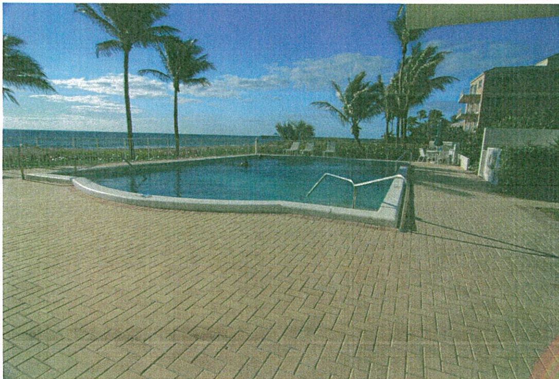
EXHIBIT 1. OVERALL VIEW OF POOL AND DECK LOOKING SOUTHEAST
