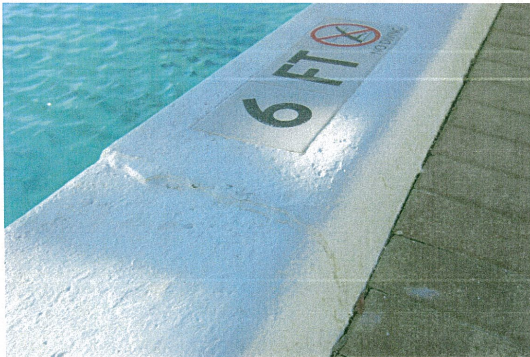
EXHIBIT 8. VIEW OF REPAIRED DISBONDED COPING STONE
